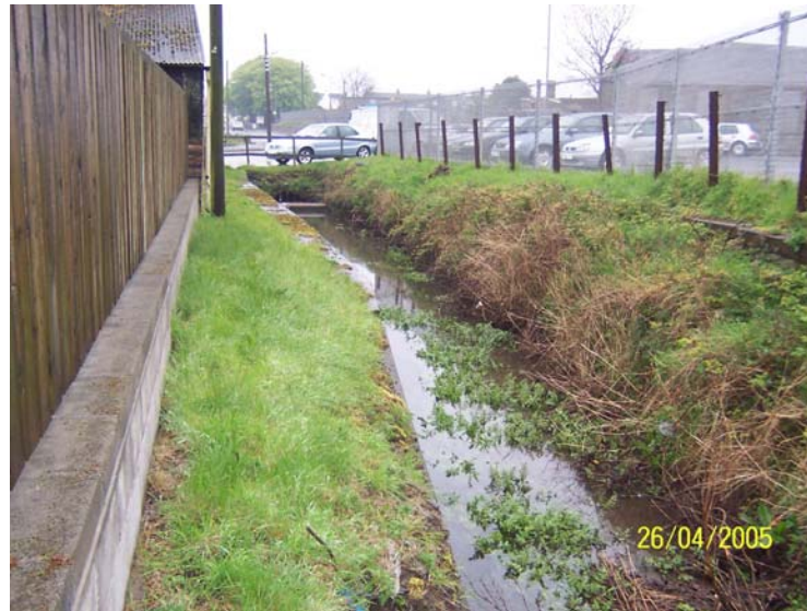
Town Burn Downstream of Railway Culvert
