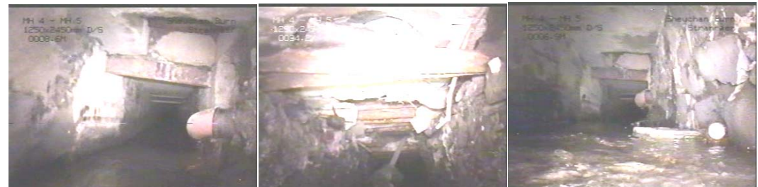
Stills from Millburn Court CCTV Survey (John Bunting, EEC - 7 July 2005)
