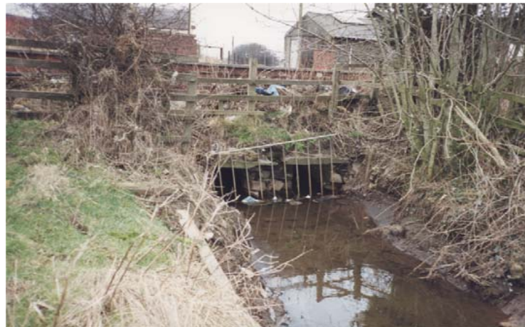
Town Burn Railway Culvert
